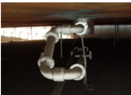
Coated carbon steel drain line arrangement.
