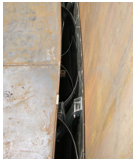
CTS1 scissor shoe plate seal, top view during installation.
