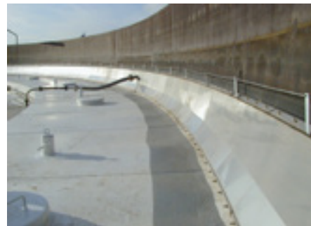
CTS20L secondary seal with direct foam injection.
