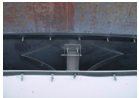
CTS1 scissor shoe plate seal during assembly.
