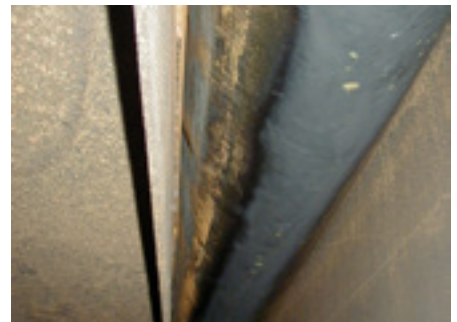
CTS7 out of service inspection, bottom view
