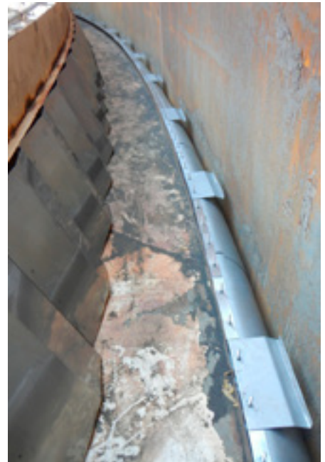
CTS30 seal during installation, top view.
